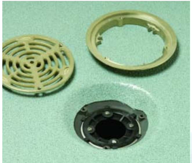
Stainless steel drain prior to fitting vinyl clamping ring
